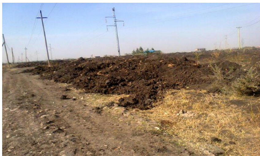
Plates 2: Deposit of Cotton soil along the road in Mavoko, Nairobi, Kenya (Researcher, 2015)
