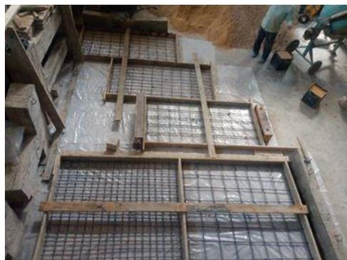
**Fig 5: Reinforcement layout of Slabs of Group I**
