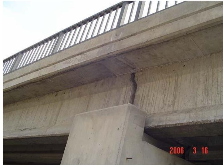
**Figure 2: A bridge with link slab after earthquake.**
