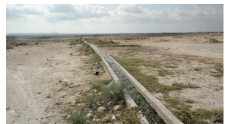
Figure 6 An overview of the Ghail Bawazir (Bawazir Stream) Canal.
